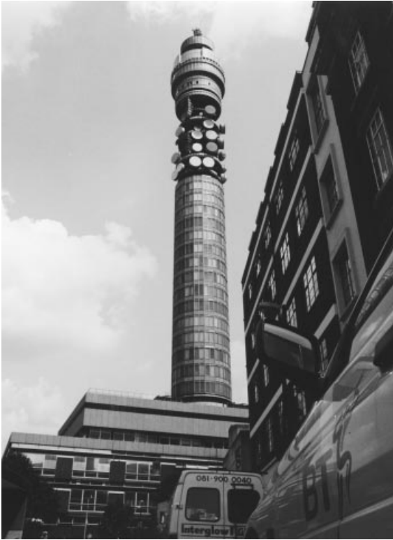
Figure 2.8 The BT telecommunications tower in London. (BT Corporate Picture Library: A BT Photograph.)
